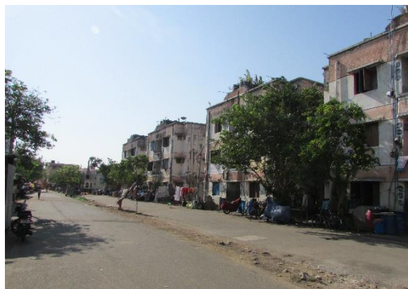
Figure 57: Cement road in Kannagi Nagar- Source: K.Hochart, April 2014
