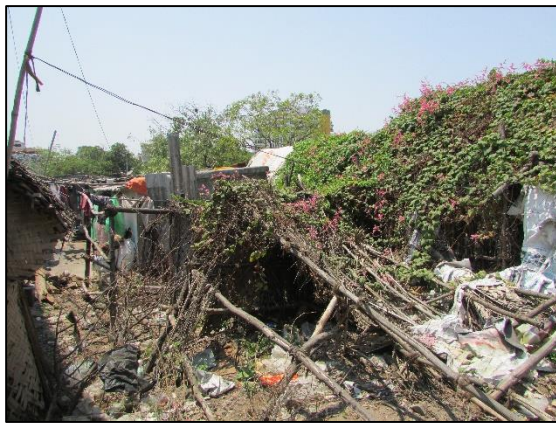
Figure 50: Huts destroyed by floods in Attur Nagar- Source: K.Hochart, March 2014
