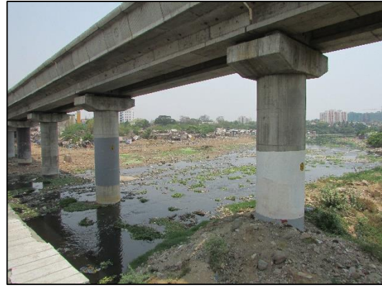
Figure 33: View of the metro bridge across Adyar River with Attur Nagar in the background – Source: K.Hochart, April 2014
