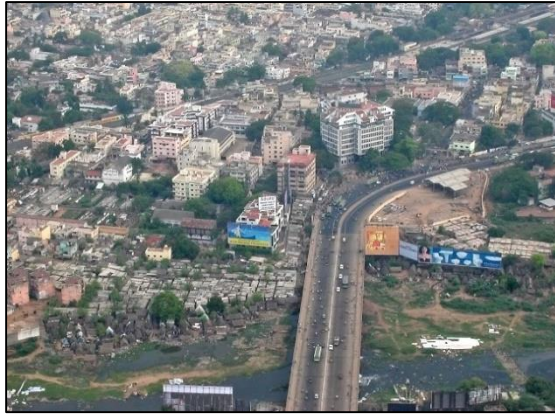
Figure 32: Aerial view of Maraimalai Adigal Bridge, previously known as Marmalong Bridge, across Adyar River in Saidapet – Source: Wikipedia, Saidapet
